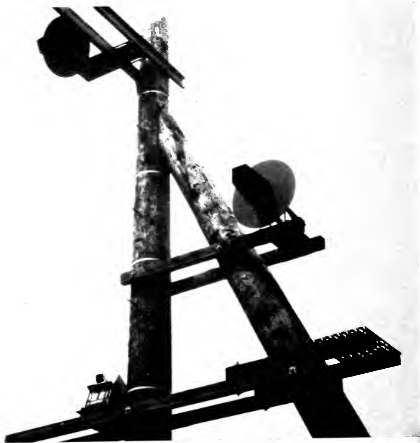
Fig. 3—Photoelectric detector of high and wide clearance.
